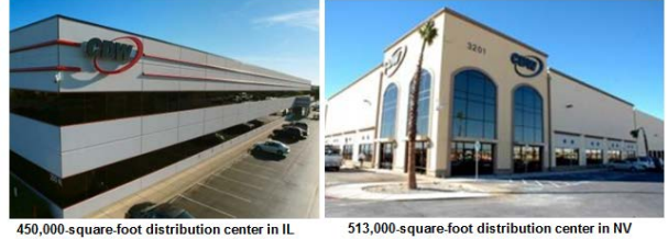
450,000-square-foot distribution center in IL
